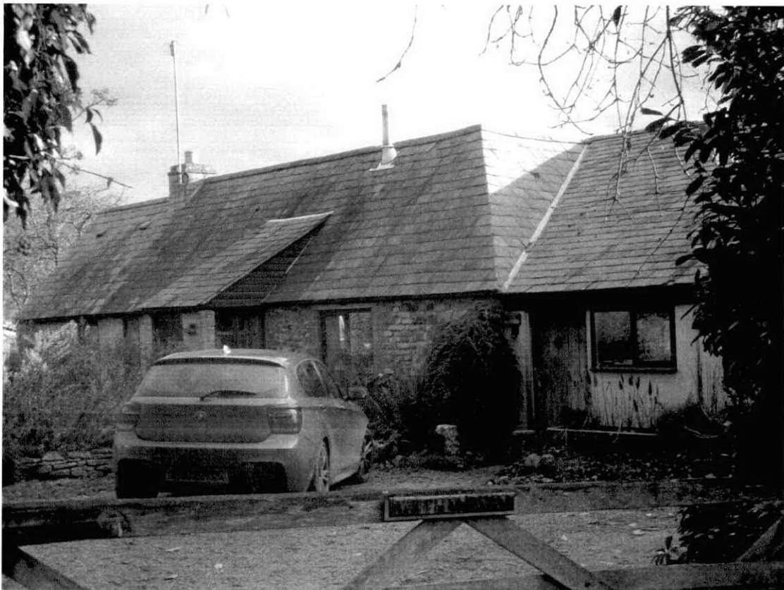
Below: Existing dwelling
